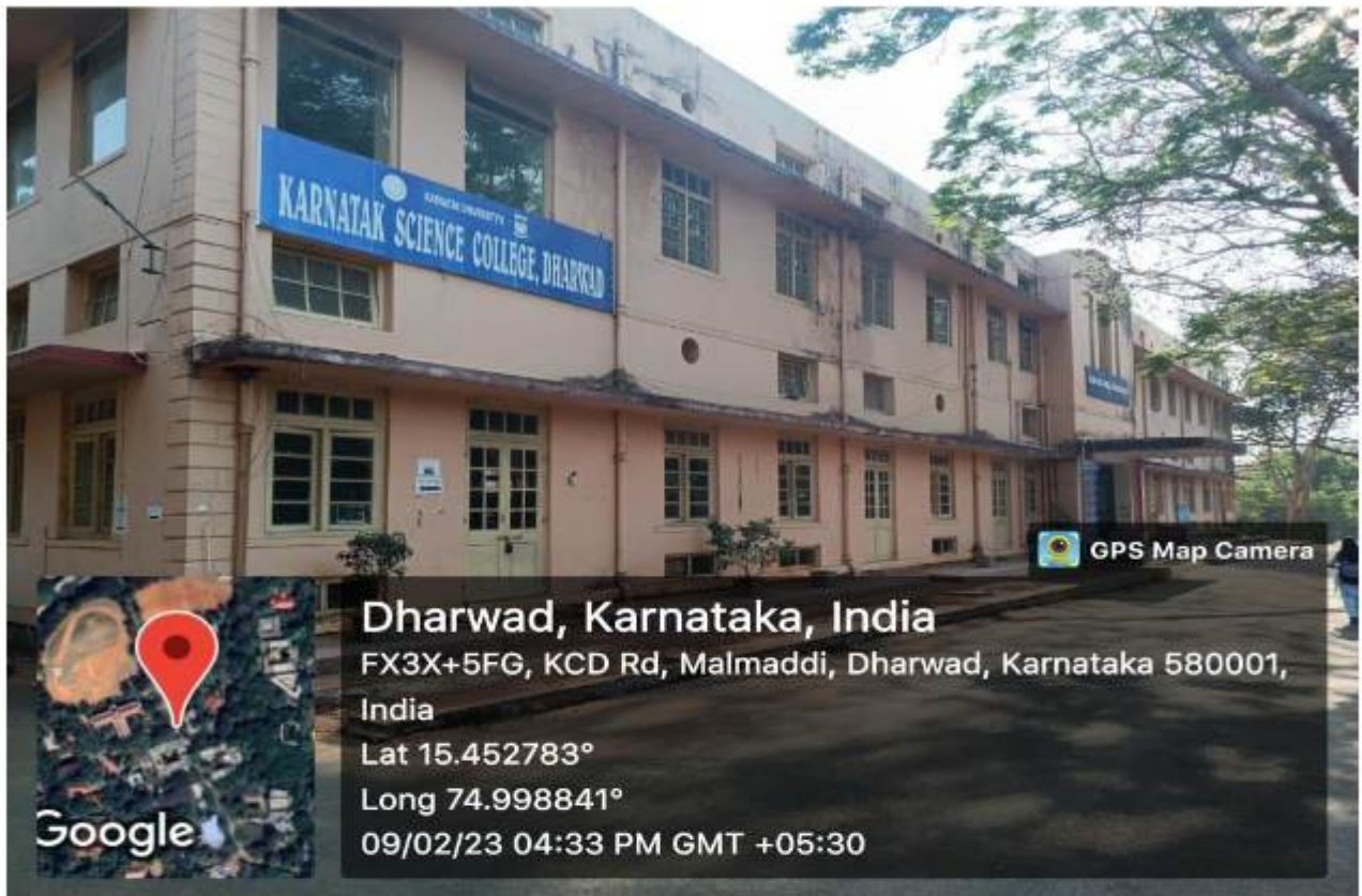
Main Administrative Block, Chemistry (UG & PG), Biotechnology, Geology & Statistics Departments.
